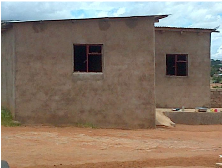
Picture 11- incomplete store house
