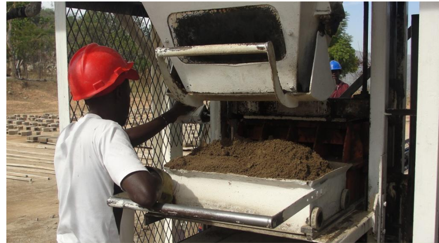
Figure 7: the mixture is being loaded on the industrial brick making machine
