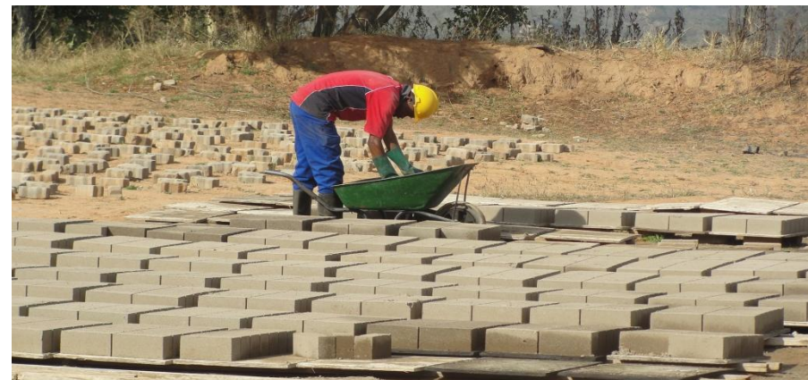
Figure 5: bricks being packed in the wheelbarrow and ready to be loaded in the truck for delivery to the local market
